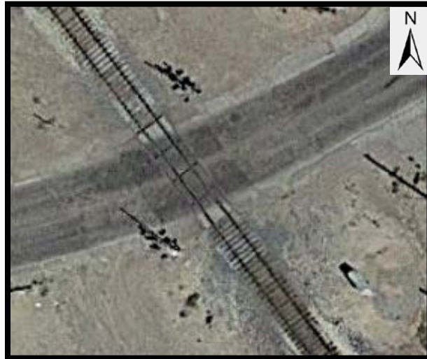
Figure C24. Rail Crossing 318 – Rio Vista Road
