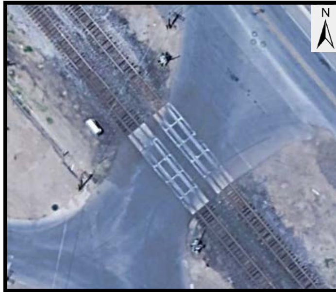
Figure C19. Rail Crossing 313 – New Haven Drive
