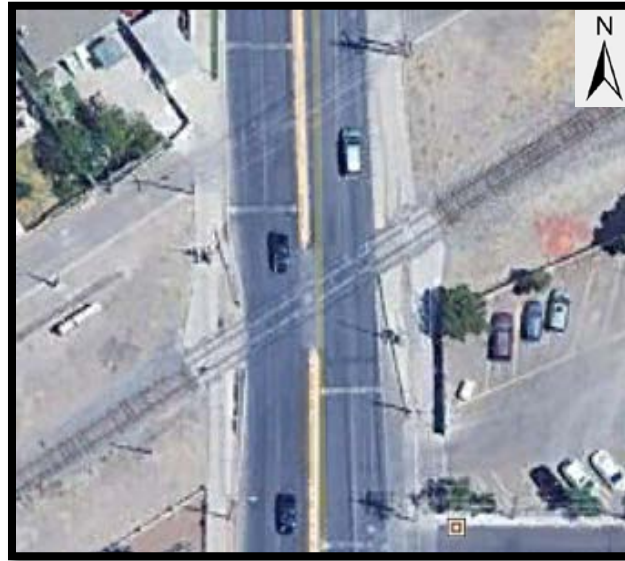
Figure C1. Rail Crossing 201 – Piedras Street
