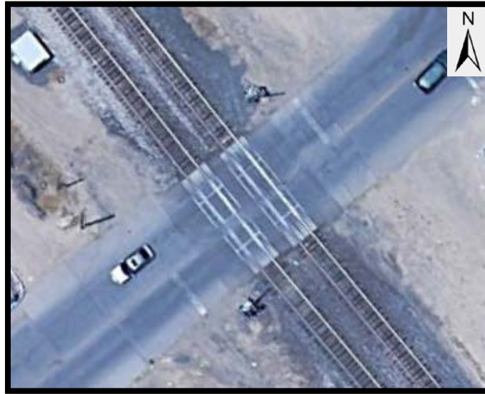
Figure C16. Rail Crossing 310 – Rosedale Street
