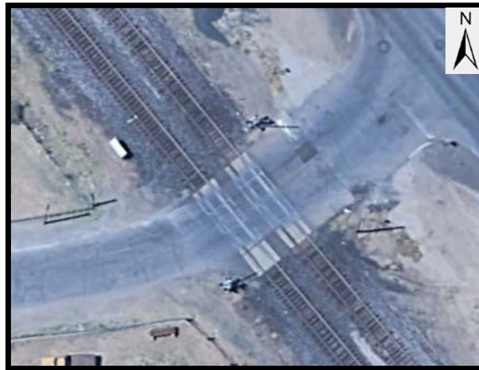
Figure C18. Rail Crossing 312 – Smith Road
