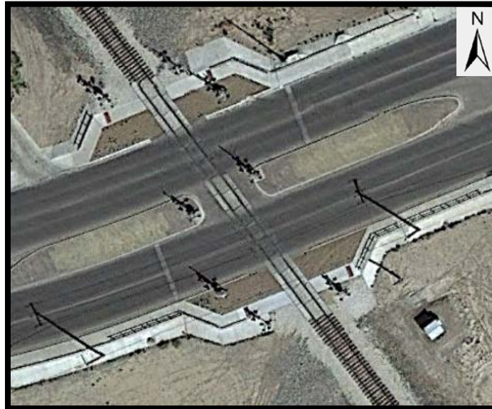
Figure C25. Rail Crossing 319 – Horizon Boulevard
