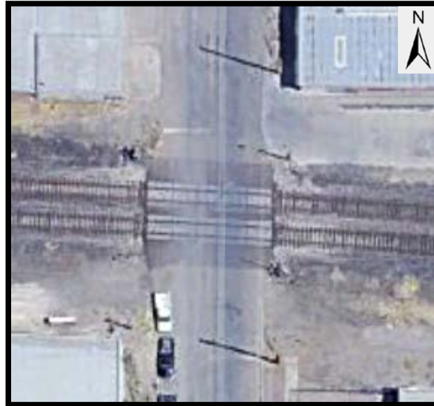
Figure C8. Rail Crossing 302 – Estrella Street
