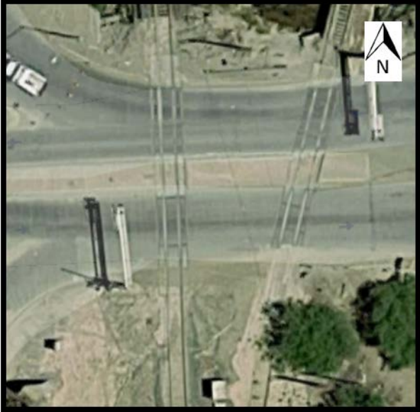
Figure A18. Rail Crossing 118 – Executive Center Boulevard
